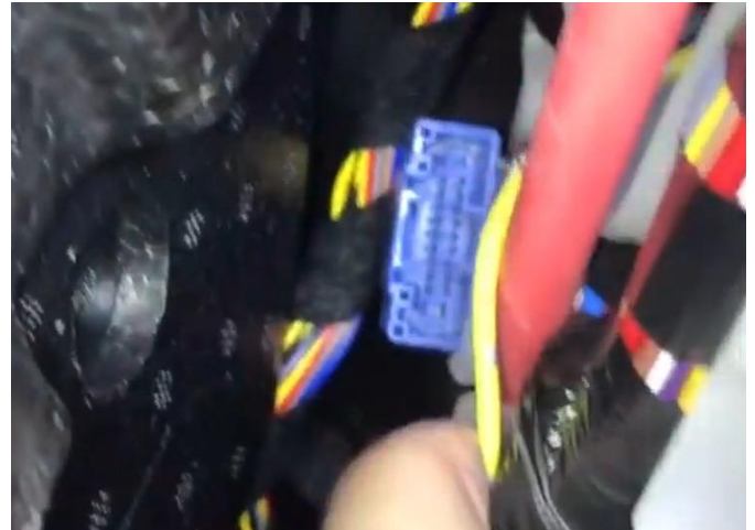
23. 拆开副驾 A 柱下方脚窝侧边饰板，找到蓝色原车协议插座，把协议线分别走线到对应的门板上 Remove the trim panel under the copilot A pillar. Find the original blue signal socket. Go through the signal wire to the corresponding door panel.
