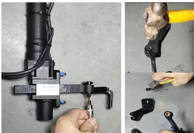
5. 用工具分开智能门执行器铰链 Use the tools to separate the chain of the actuator.
