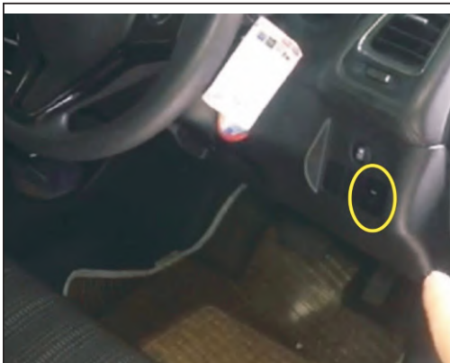
10. Installation before we switch (small lamp line by central control desk lamp line)
