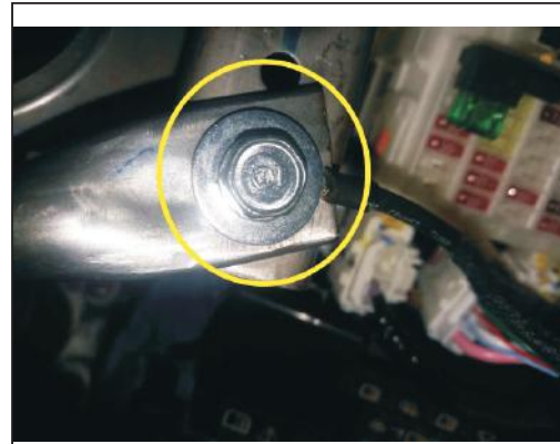
9. Found in power in front of the ground, the ground connection
