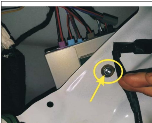
19. The installation position and control box, with our screws and washers
