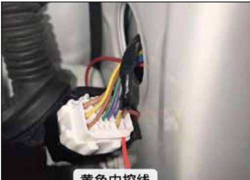
8. At B pillar connected with central control wire
