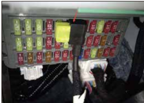
6. Power access at the original car driver compartment
